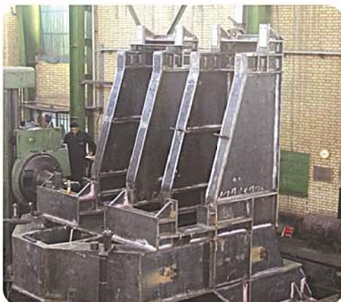
Complex Furnace Roof Lifting (KSC)
