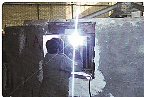
Welding mill ring gear - Chadormalu iron ore company
